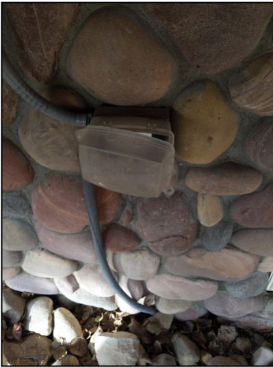
Outlet under the front deck had no power
