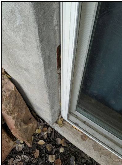
Lower level windows are not sealed well around the edges
