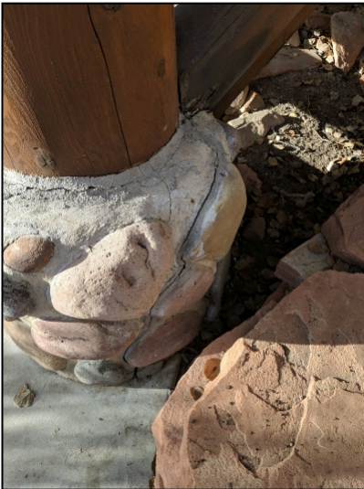
Mortar maintenance advised on stonework
