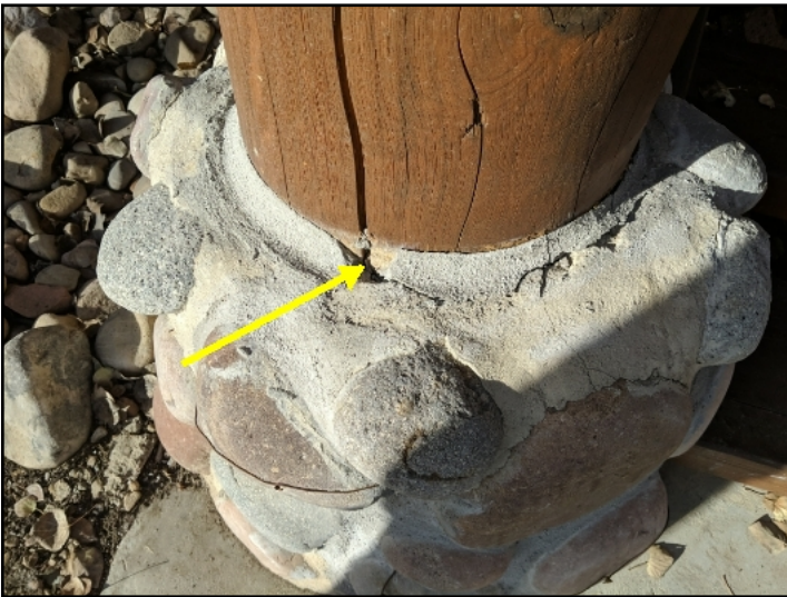
Posts have water damaged wood where they meet the stonework
