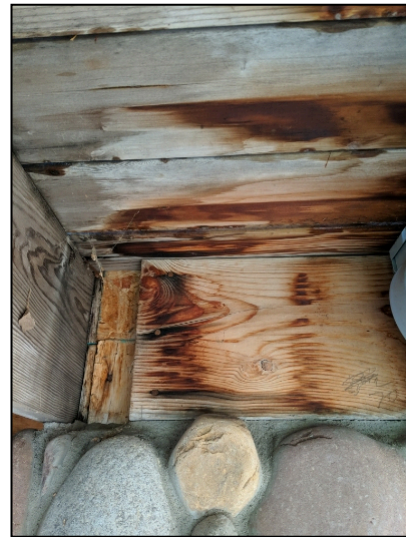
Exposed OSB and lack of flashing under front deck
