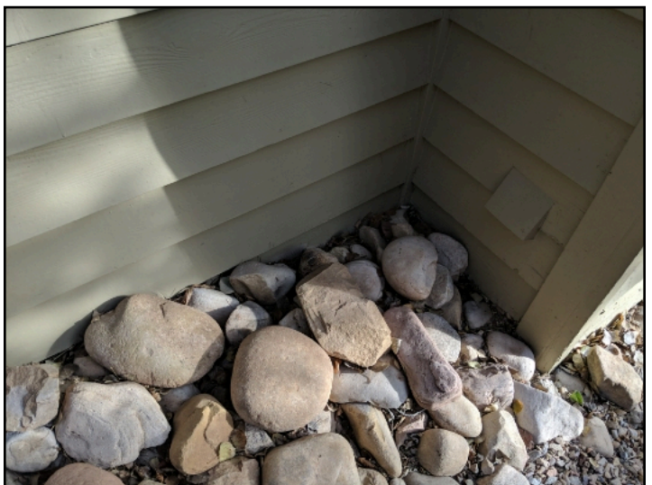
Wood in contact with Earth in a few areas
