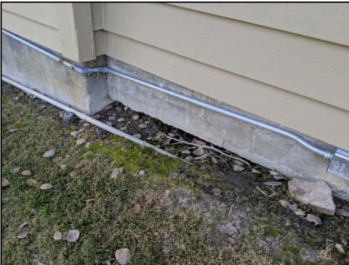
Hollow under storage area slab
